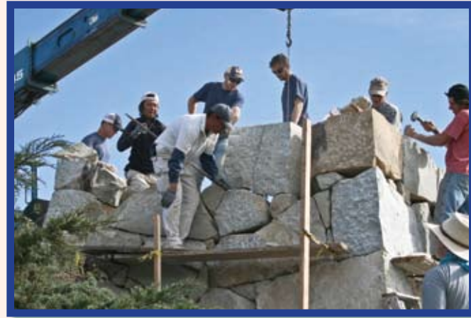
Ojai Quarry Stone donated the valuable stones for creation of Ventura's Grant Park rock work. This phone taken, January, 2010. Suminori Awata (15th generation stonemason in the Anoh tradition of Japan) designed and with his assistant shifts a boulder on the west side of the rampart with a prybar, while the crane cable holds the rock a little up. Suminori knocked one melon-sized chunk off this boulder, with one perfect sledgehammer blow. The mason at the right chisels to shape the rock placed an hour before - he was skilled enough to be able to chisel without protective eyewear.
